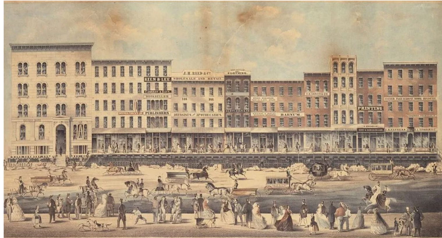
Raising a block of buildings on Lake Street, Chicago, in 1857 Chicago Historical Society/Wikimedia Commons.
